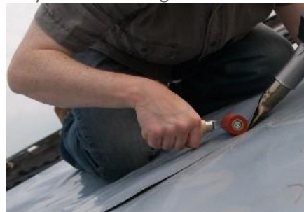
Single Ply Roof Welding
