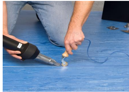
Vinyl Floor Welding
